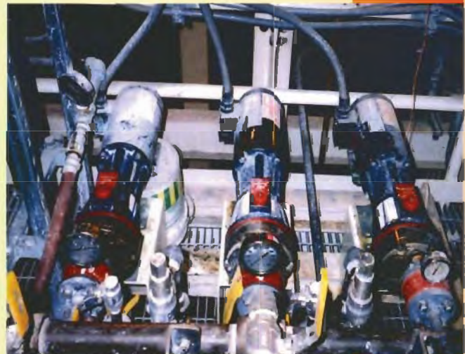
Flue Gas Desulfurization
