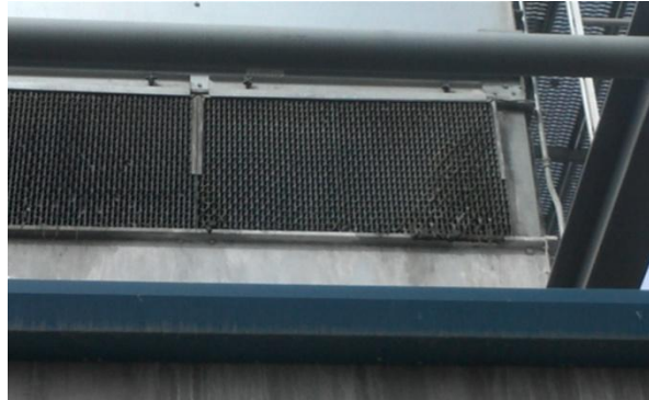
3 weeks later - Scale is gone and bio growth is being eradicated.
